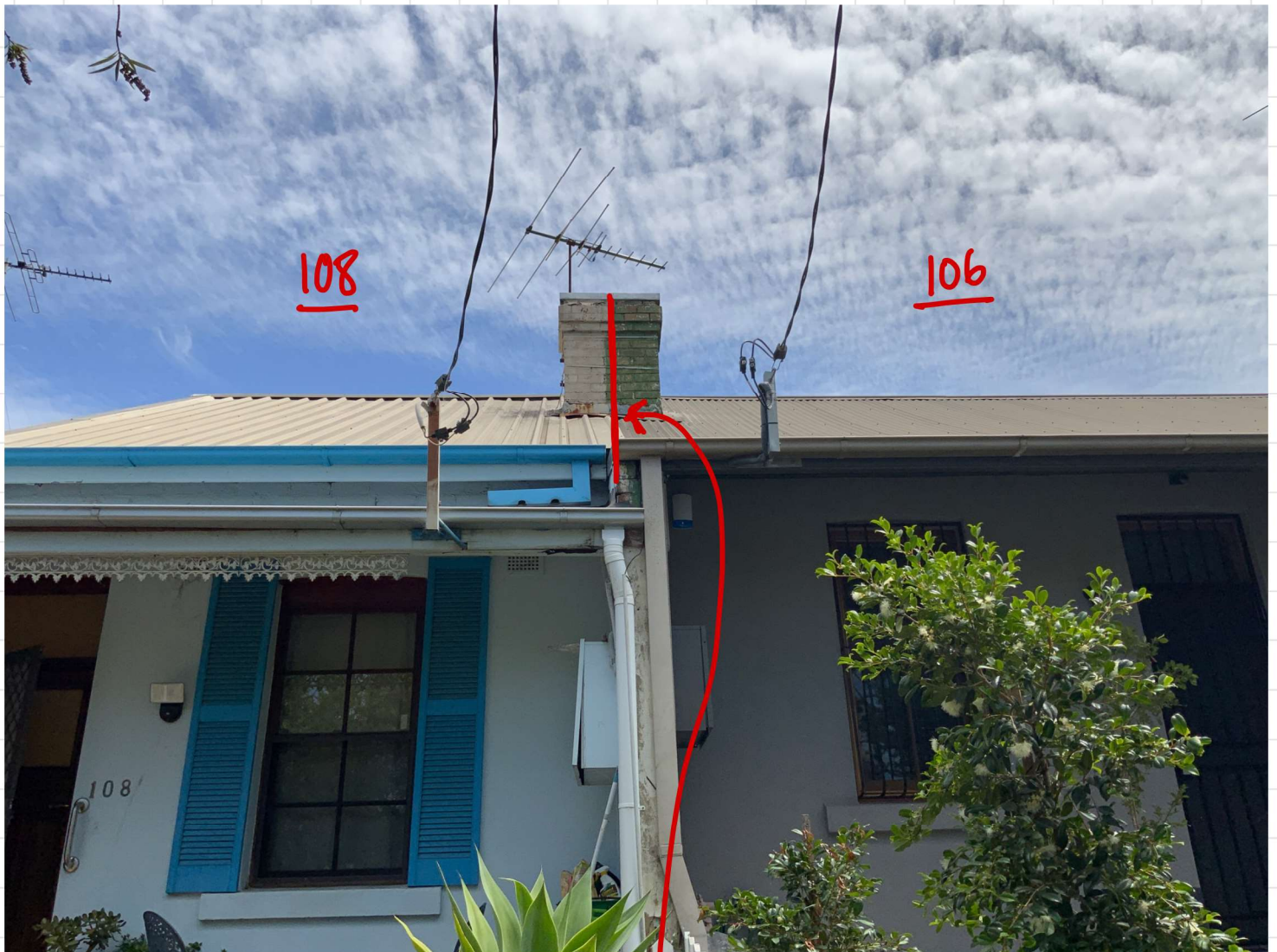
Photo ④ - Front Chimney at 108/106
